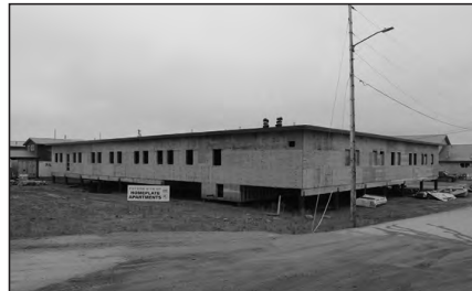
HOUSING —The construction of the HomePlate apartments is progressing. Northrim Bank donated $10,000 toward the project.
